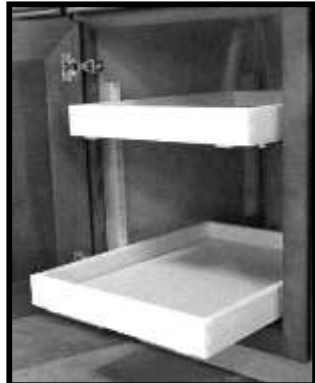
TWO ROLLOUTS INSTALLED
